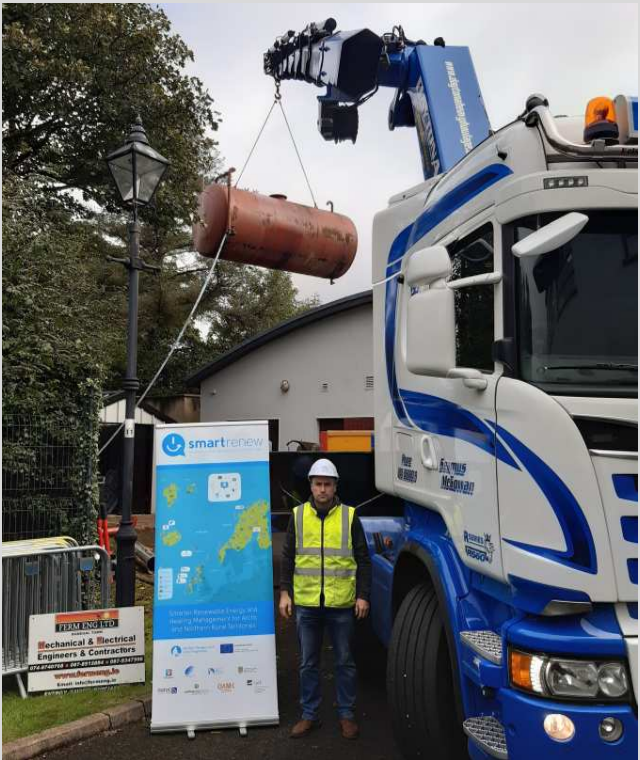
Oil Tank Removal
